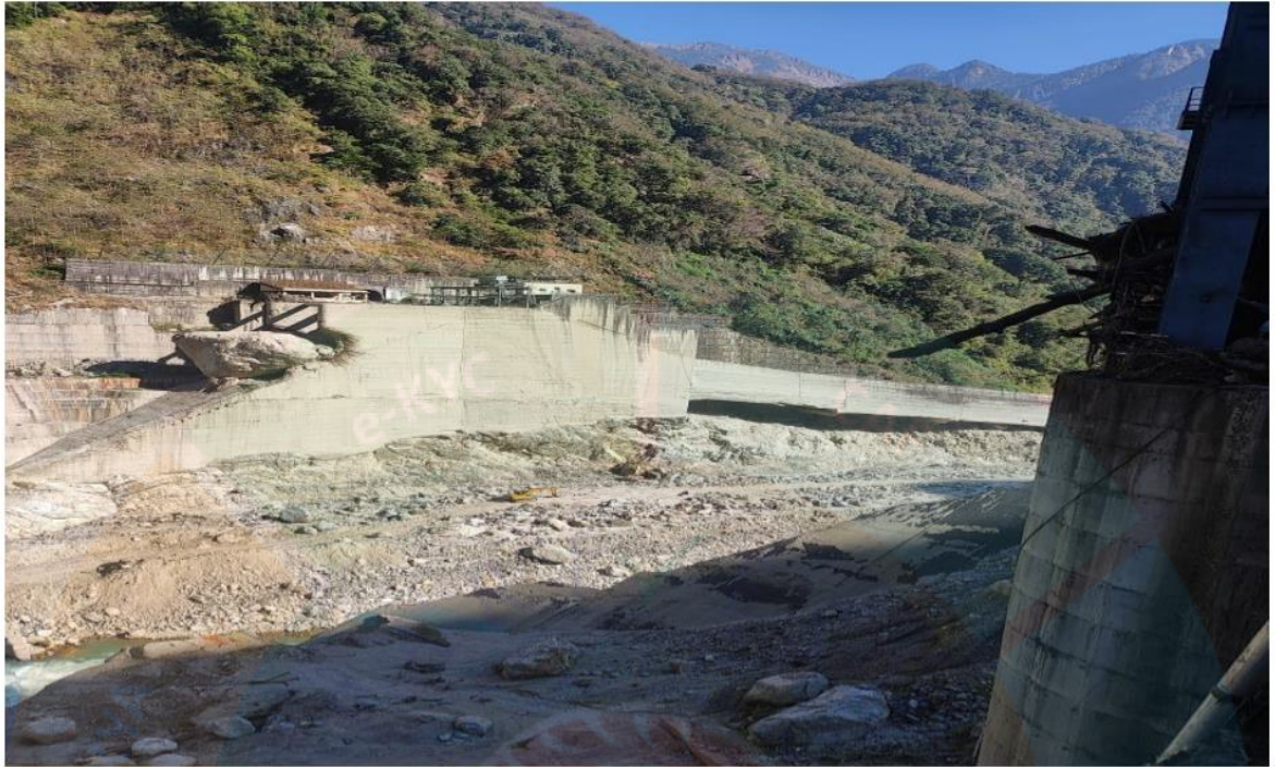
Fig: Remnant of washed away CFRD
