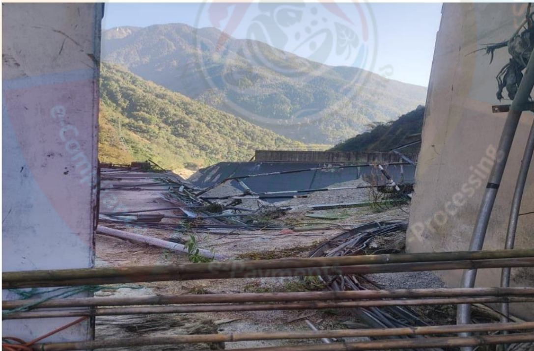
Fig: Damaged chute spillway
