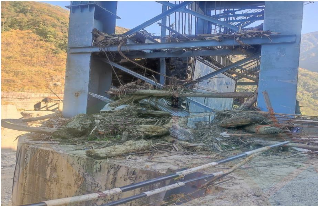
Fig1.Damaged Gate Structure
