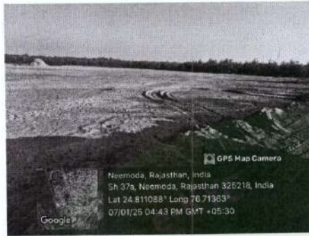
Existing Ash Pond
