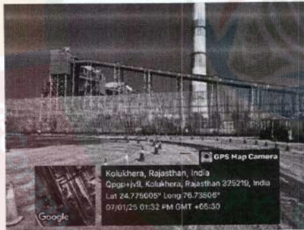
Conveyor Belt and Wind Barrier
