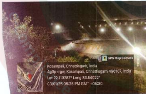
Backfilling of void by fly ash in nearby mine (with combination of 3:1 fly ash and OB material)
