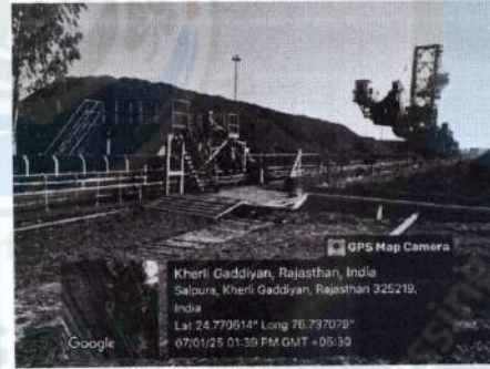
Coal Stock Yard
