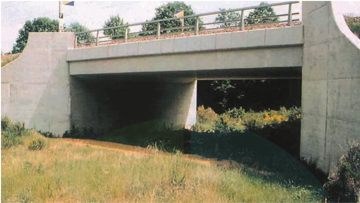
Figure 9: Example of a underpass below highway with good openness index and suitable for the movement of large mammals as well as other wildlife species of the landscape. (Google images).
