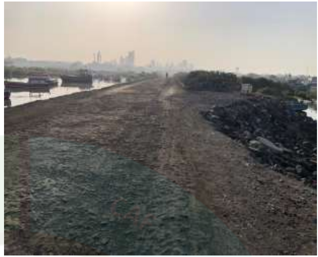
Approach Road for Litrage Jetty.
